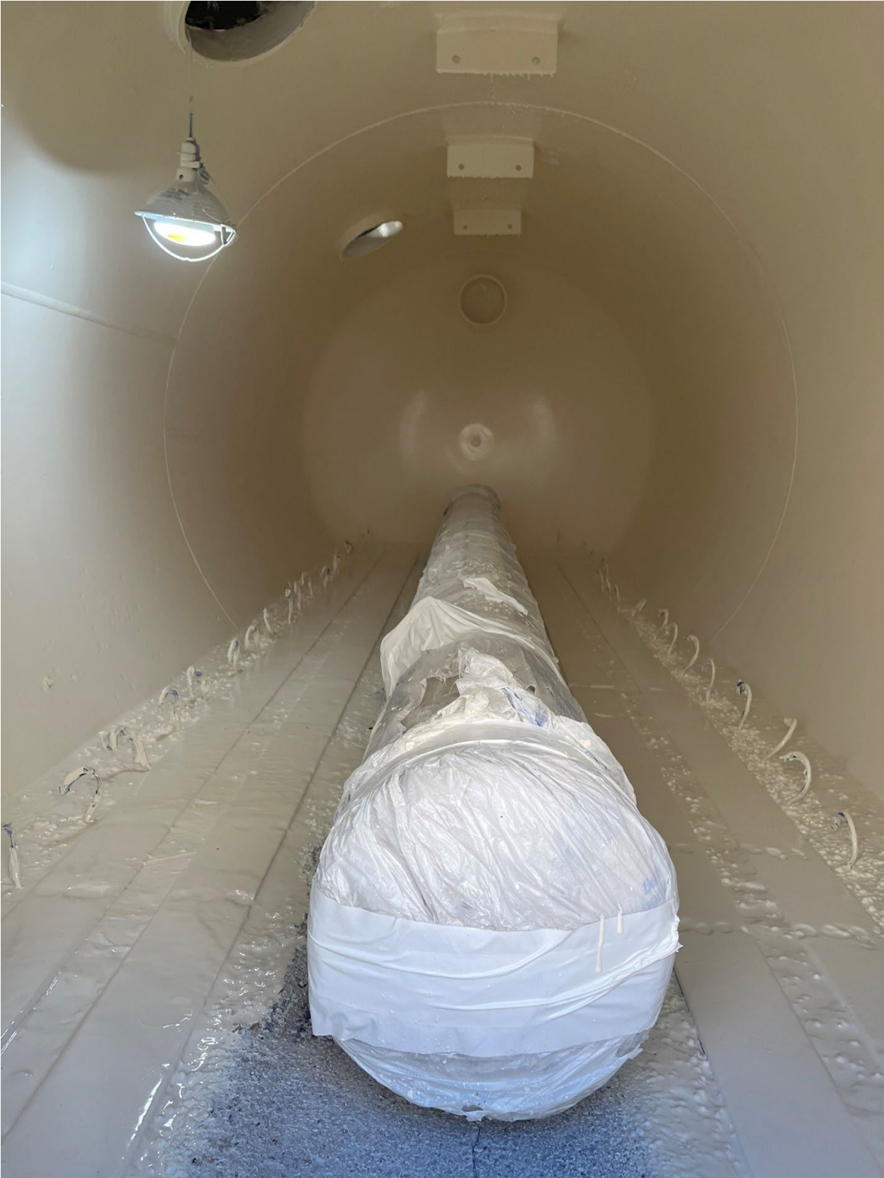
Filter Tank Completed,
